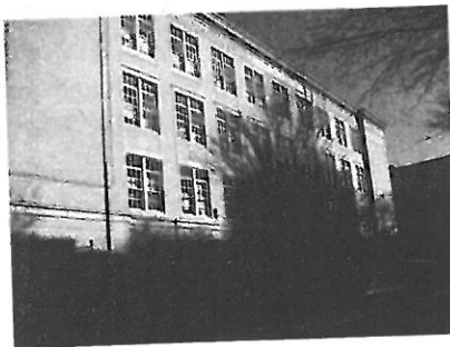
FIGURE 12.6. Public School 94 and 3508 Kings College Place (the Preds' building).
